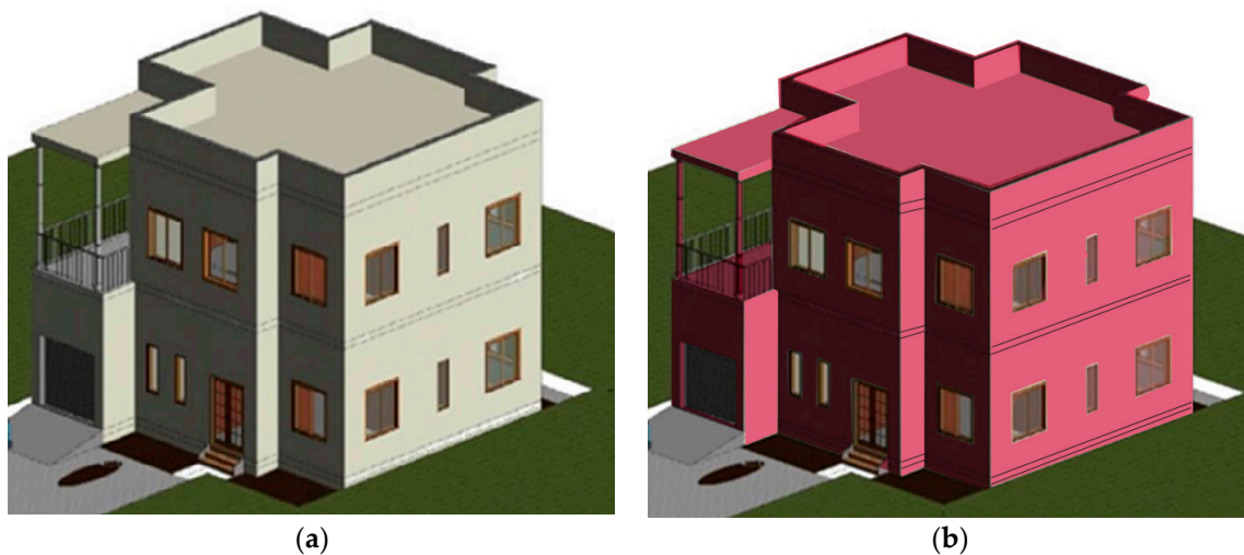
Figure 9. (a) Two story residential building with common coatings. (b) Two story residential building with low-brightness and high-reflective coatings.
