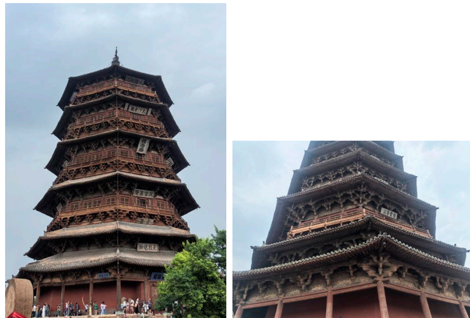
Figure 2. On-site photos of the Sakyamuni Pagoda of Fogong Temple. Source: Photo by Xuejiao Li.
