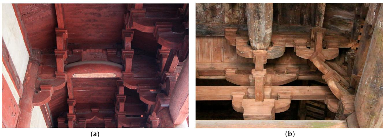
**Figure 5.** Clues for the form of palatial hall frames in eastern Fujian: beams intertwine with bracket sets to support the ceiling: (a) The front corridor of the main hall in Hualin temple; (b) the Song structure of Chen Taiwei Palace. Photography by authors.
