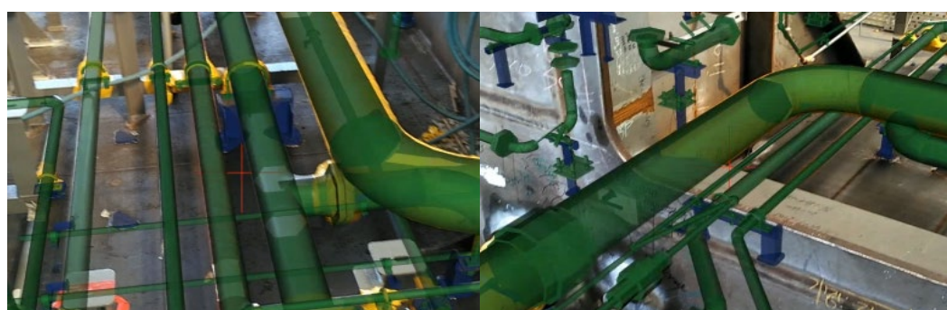
Figure 15. Examples of accurate AR scene generation. The pipe and pipe support CAD models are augmented very precisely on the real objects.
