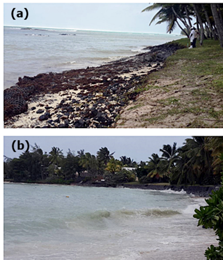
Figure 12. (a) Damaged beach with exposed rock-filled gabion baskets after cyclone Berguita in January 2015. (b) The dominant wave at the study site drives a net transport to the west.
