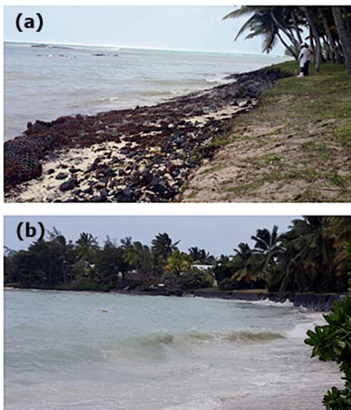
**Figure 12.** (a) Damaged beach with exposed rock-filled gabion baskets after cyclone Berguitta in January 2015. (b) The dominant wave at the study site drives a net transport to the west.
