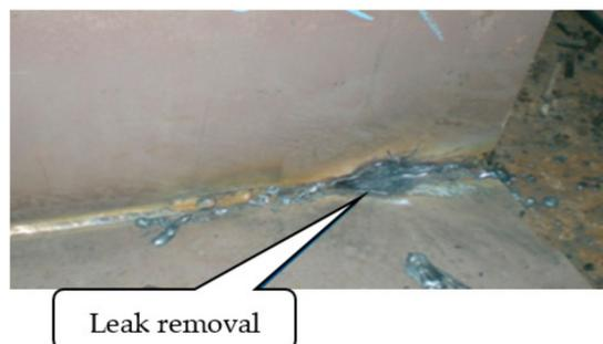
**Figure 18.** Piece leak removal.
