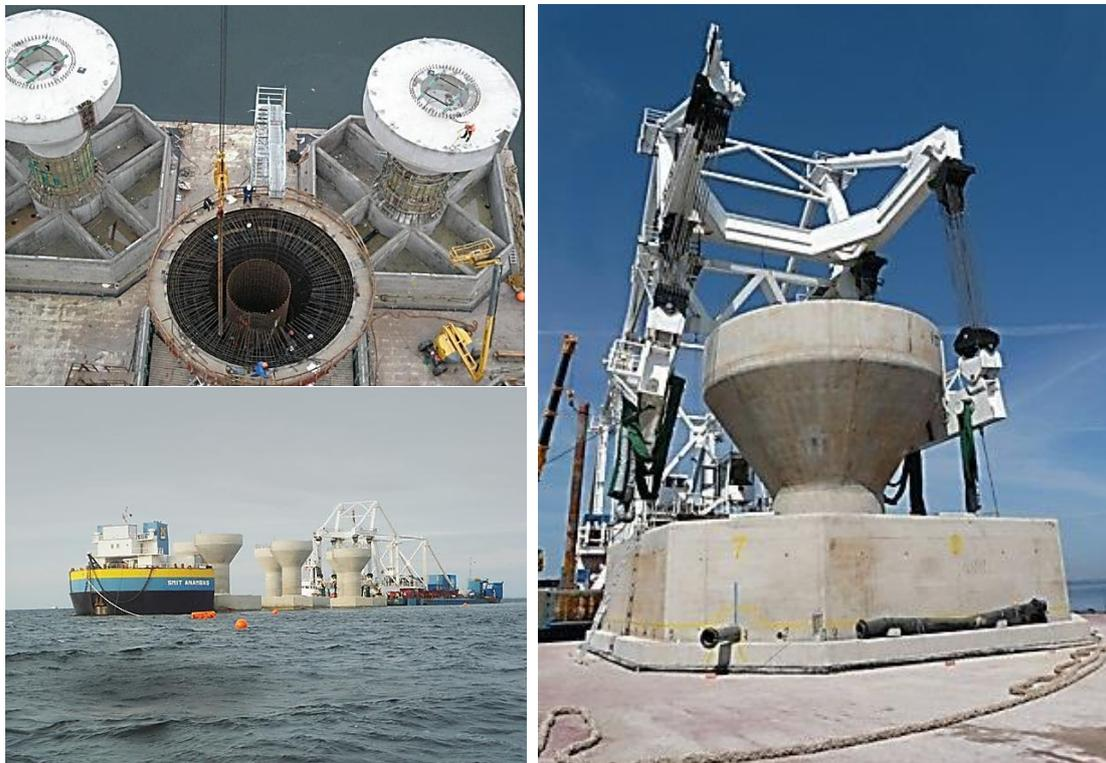
Figure 5. Rødsan II (or Nysted II) offshore wind farm foundations, reproduced from [22], with permission from Aarsleff, 2019.
