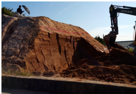
Figure 6. Slope cutting by a backhoe.
