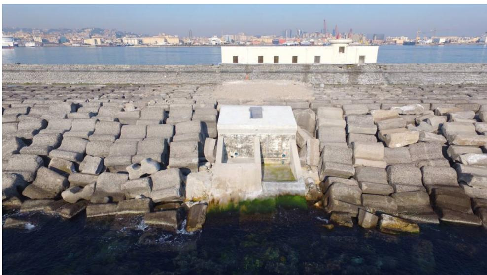
**Figure 2.** The 6 m wide OBREC prototype operating at the Port of Naples (Italy), integrated into the main breakwater with an ANTIFER-type armour layer.
