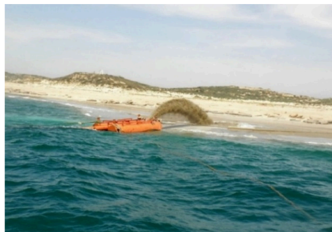
Figure 12. Nourishment rainbowing operation via discharge pipe, north of Ashdod Port, May–August 2011. Photograph courtesy of EDT Marine Construction (Figure 2 in [22]). Used with permission.
