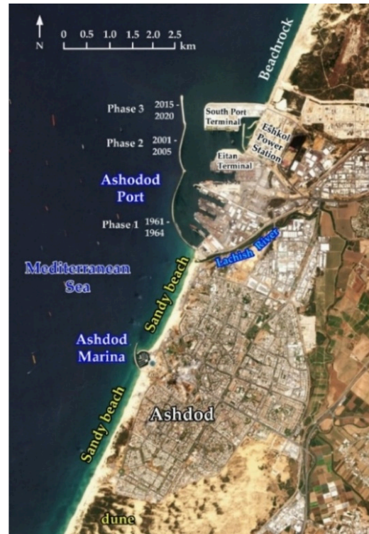
Figure 7. Ashdod Port in 2022, one year after completion of its second expansion. The Eshkol Power Station cooling-water basin is enclosed within the expanded port area between the Eitan Terminal and South Port while continuing to function as the cooling-water facility of the adjacent power station. Background image: Copernicus Sentinel-2 L2A, acquired on 20 May 2022. Credit: European Union, contains modified Copernicus Sentinel data 2022, processed with Sentinel Hub.
