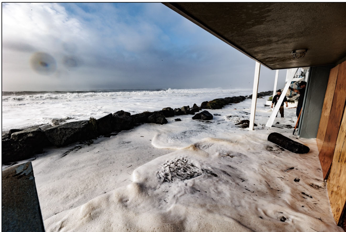
Figure 8. Flooding of beach-level homes on Rio del Mar's Beach Drive from very large waves at high tide on 2 January 2024 (Kevin Painchaud- Lookout Santa Cruz).
