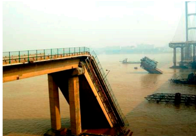
Figure 1. Collapse of Jiujiang Bridge under errant ship impact in Guangdong Province, China (2007).
