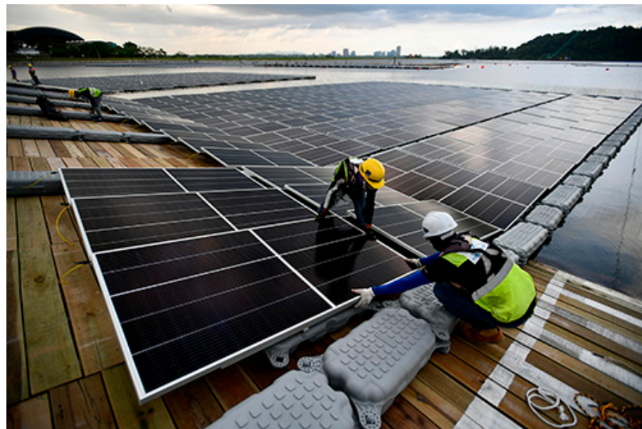
Figure 7. Workers are installing photovoltaic modules on floating modules waiting to be transported to the designated location [86].
