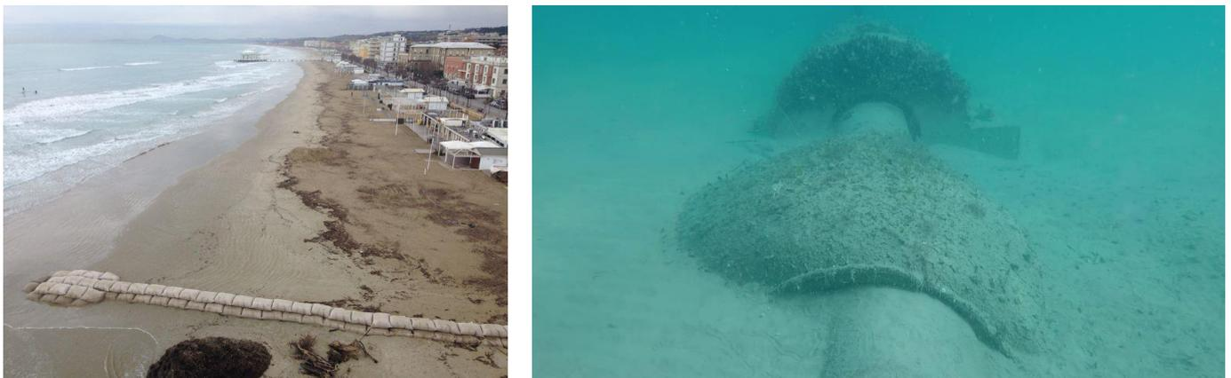
**Figure 2.** Application of “Stopwave” as temporary groin in Senigallia, Italy (**left panel**) or as pipeline protection (**right panel**).
