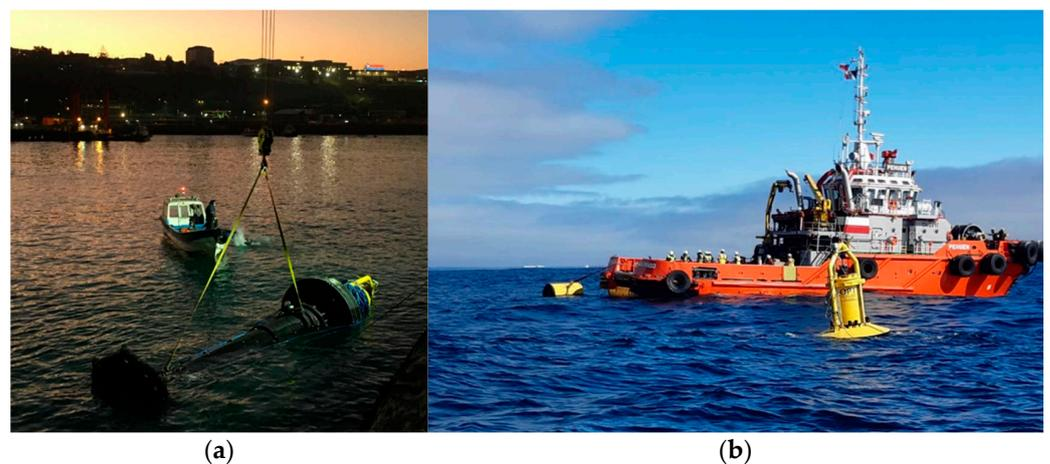
**Figure 7.** (a) Lowering of the PB3 PowerBuoy into the water at San Antonio Port. (b) PB3 PowerBuoy deployed at its final position in Cartagena Bay.
