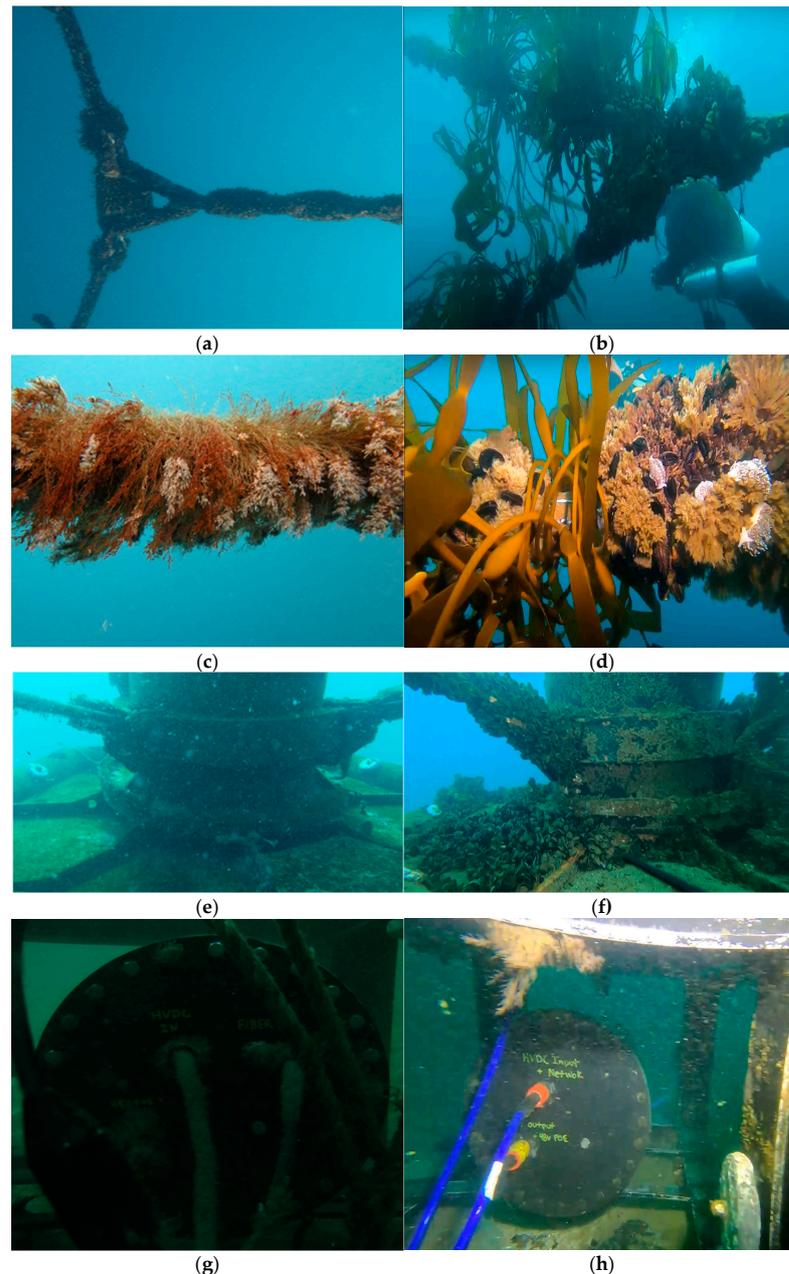
**Figure 12.** Images taken during two inspections 3 and 15 months after installation, including a triple mooring connector between the PB3 and the auxiliary buoys at a depth of 5 m in July 2021 (a) and July 2022 (b). Holding rope in July 2021 (c) and July 2022 (d). Balance plate in July 2021 (e) and July 2022 (f). First junction box at a depth of 34 m in July 2021 (g) and July 2022 (h).
