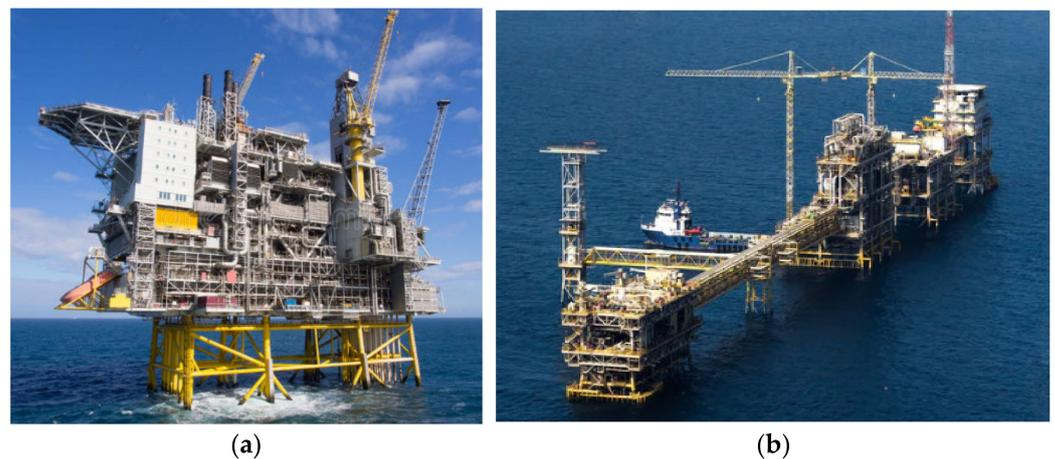
**Figure 4.** Typical platforms showing (a) conventional jacket platforms and (b) bridged fixed jacket platform on Zuluf oil field in Arabian Gulf, offshore northeast Saudi Arabian coast, with the water depth of about 40 m (Image (b) Courtesy: Saudi Aramco).
