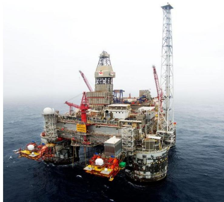
Figure 17. Heidrun Tension Leg Platform (TLP). (Courtesy: Statoil.).
