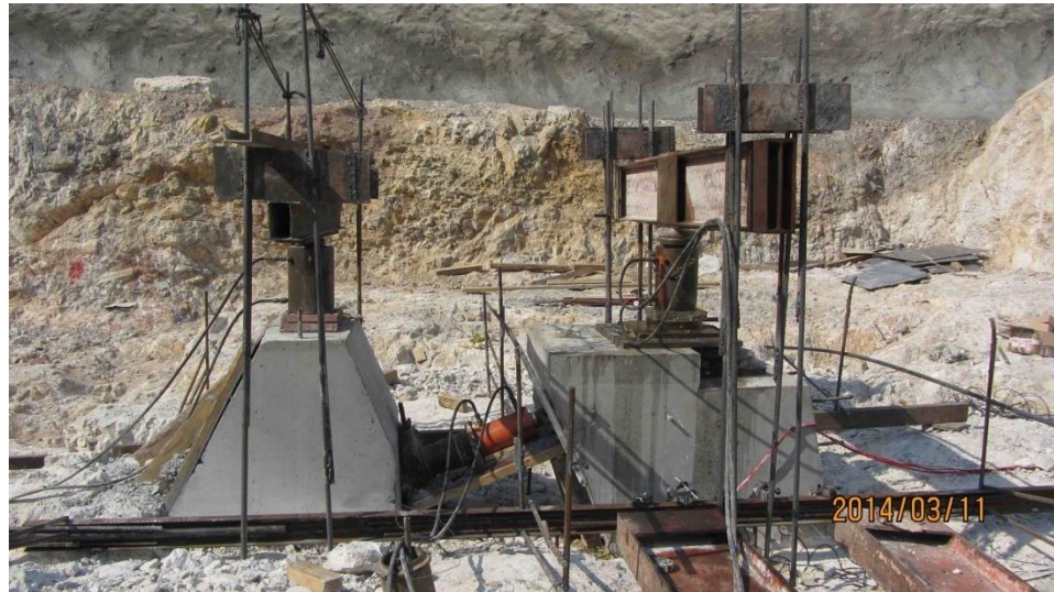
Figure 6. The in-situ scale model test of the bridge anchorage.
