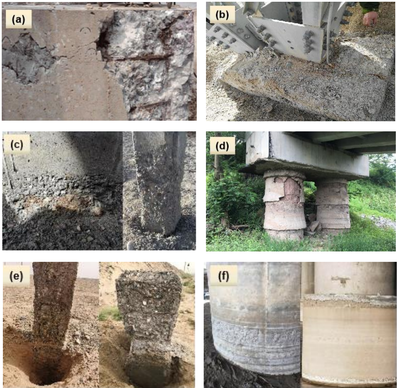
Figure 5. Deterioration of reinforced concrete (RC) structures due to saline-soil corrosion in different areas of China: (a) RC stand column in a coastal area of Tianjin city, China [70]; (b) transmission tower RC foundation in Qarhan area, Qinghai Province, China [61]; (c) RC stand column in Qarhan area, Qinghai Province, China [61,65]; (d) RC bridge pier of Tarim River, Xinjiang, China [66]; (e) RC boundary monument in Hotan area of Xinjiang, China [66,68]; (f) RC bridge pier in Hetao area of Inner Mongolia, China [71].
