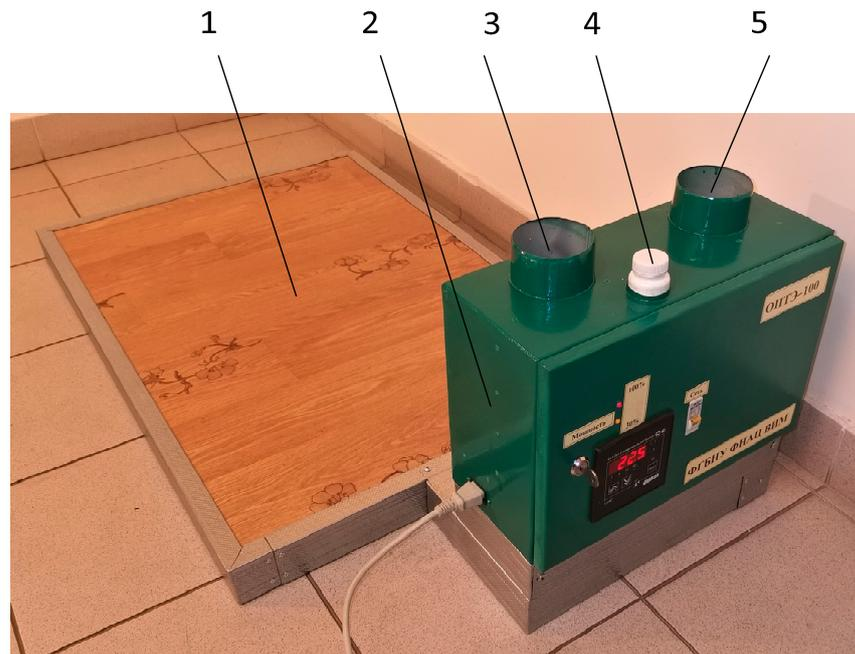
**Figure 4.** Outlay of the heating panel: 1—floor-mounted heating panel; 2—control panel; 3—air intake; 4—heat-carrier tank; 5—exhaust air pipe.
