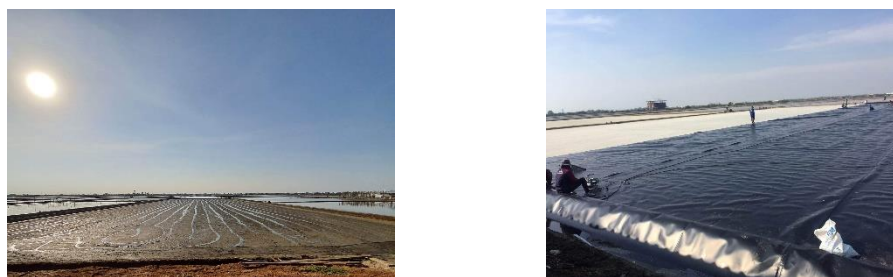
Figure 2. Traditional technology (Left) and HDPE-geomembrane-lined pond (Right).
