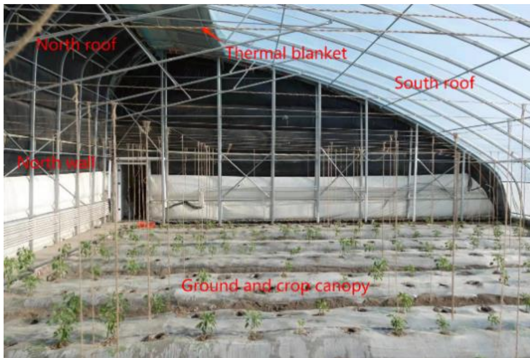
Figure 2. Internal views of CSG.
