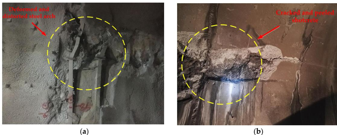
Figure 12. (a) Deformed and distorted steel arch and cracked shotcrete; (b) cracked and peeled shotcrete.
