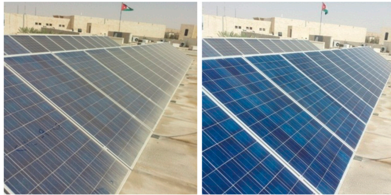
Figure 1. A 7.98 kWp photovoltaic (PV) system installed at the Hashemite University, Zarqa, Jordan before and after cleaning (all 28 modules in the foreground were cleaned manually on 24 September 2014. Modules in the background are not part of this study).
