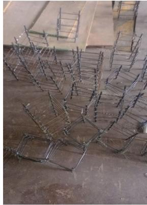
Figure 2. Assembled steel cages.
