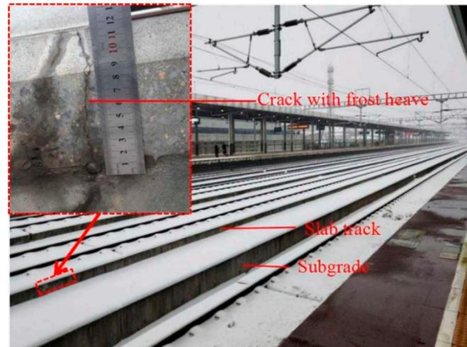
**Figure 1.** Slab-track cracks with frost heave.
