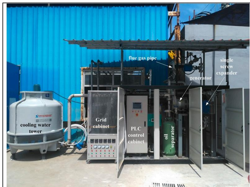
**Figure 26.** Demonstration project of ORC system used for the waste heat recovery of flue gas from a gas-fired internal combustion engine generator unit.
