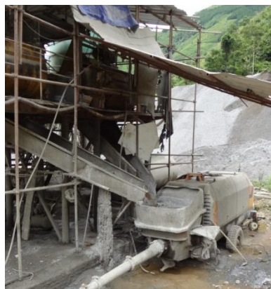
Figure 2. Pumping SCC into the working space.
