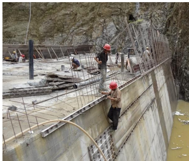
Figure 4. Poured dam body by RFC.
