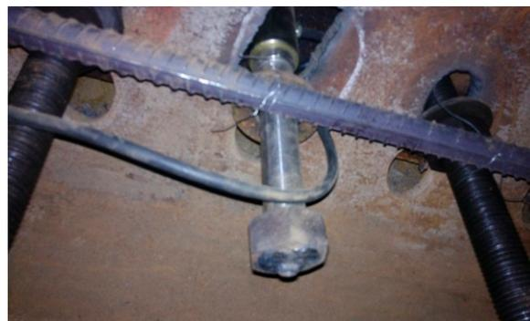
Figure 15. Installation of monitoring sensors.
