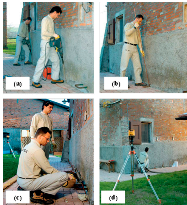
Figure 3. Stages of the process: (a) Drilling, (b) Introduction of the injection pipes, (c) resin injection head, (d) laser level to control lifting.
