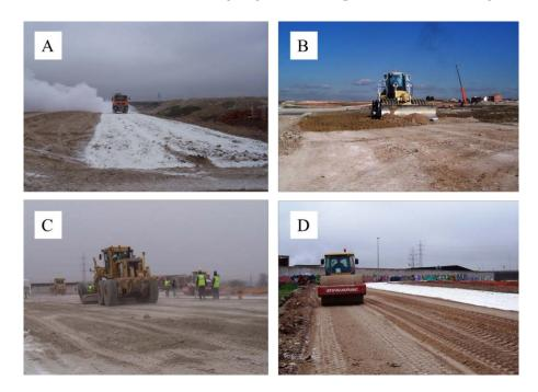
**Figure 7.** Embankment execution procedure. (**A**) Extender line on the dry soil; (**B**) mixed with lime and clays; (**C**) profiling motor grading layer; (**D**) compacting process.
