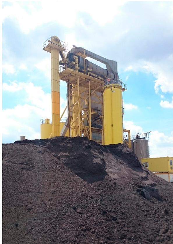
**Figure 1.** Asphalt plant with a reclaimed asphalt pavement (RAP) drum on the top and view of the RAP pile.
