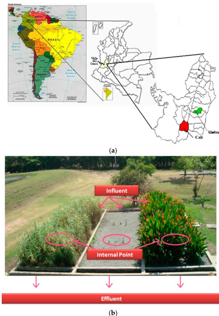
**Figure 1.** (a) Location of the pilot scale; (b) pilot scale horizontal subsurface flow constructed wetlands used in this study.
