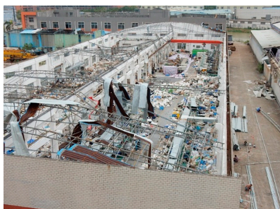
Figure 3. Mainframe collapsed during the typhoon event [6].
