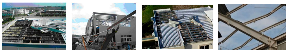
Figure 1. Failure of cladding-fastener connections.
