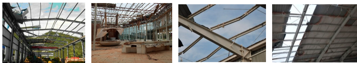
Figure 2. Buckling of Purlins under the wind uplift loadings.
