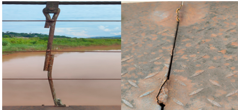
Figure 11. On-site Inspection Photos.
