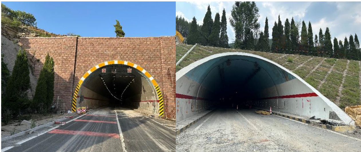
(b) Tunnel Portal
