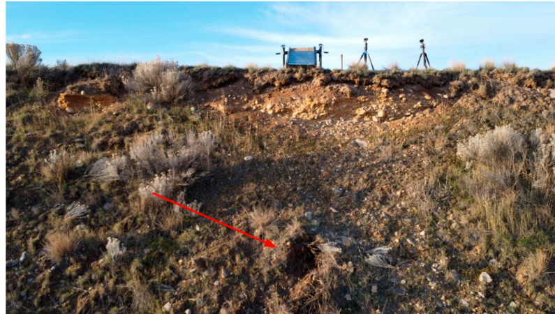
Figure 8. Scar on Slope from Block Impacts. Red arrow indicating the location of impact scar on the soil slope.
