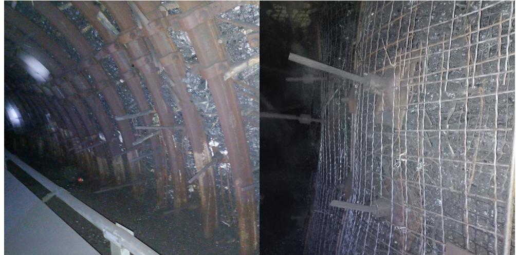
Figure 13. The real picture of the 3315 return roadway after closed opening.
