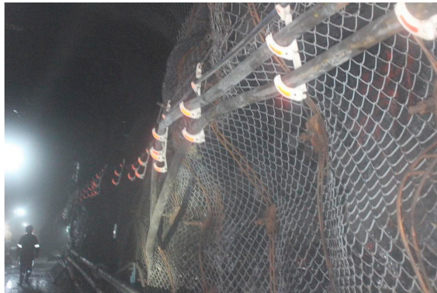
Figure 14. In situ view of the supported roadway.
