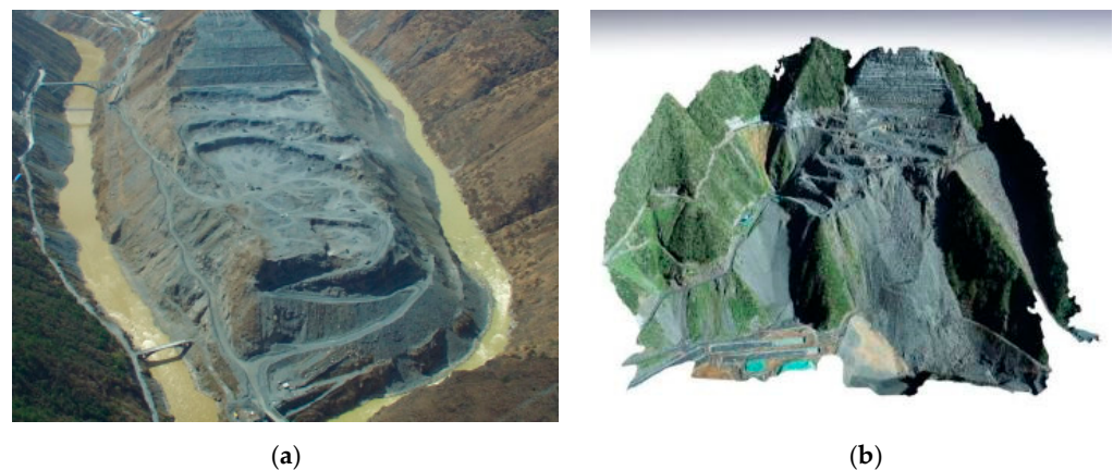
Figure 11. The grading yard (a) Lianghekou (b) Wazhigou.
