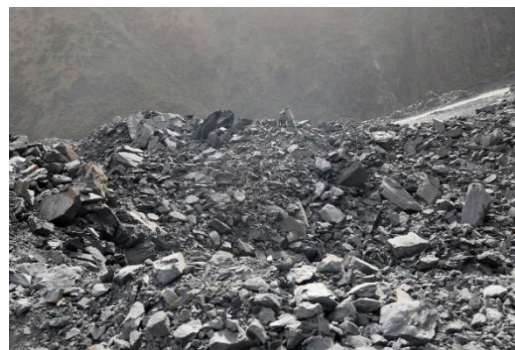
Figure 12. Typical blasting on site.
