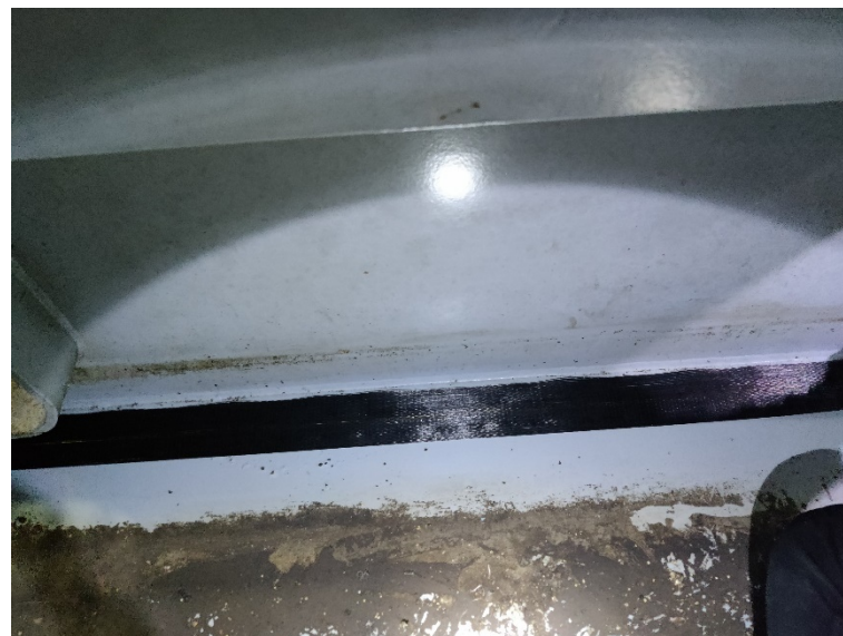
Figure 4. Real picture of the installation site.
