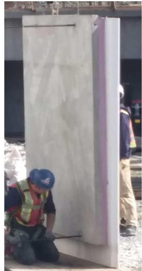
Figure 7. Details of a panel's embeds from the shop drawings designed without computational optimization ( left ); workers adjusting the panel embeds on-site due to the misalignment with the receiving embeds ( right ).
