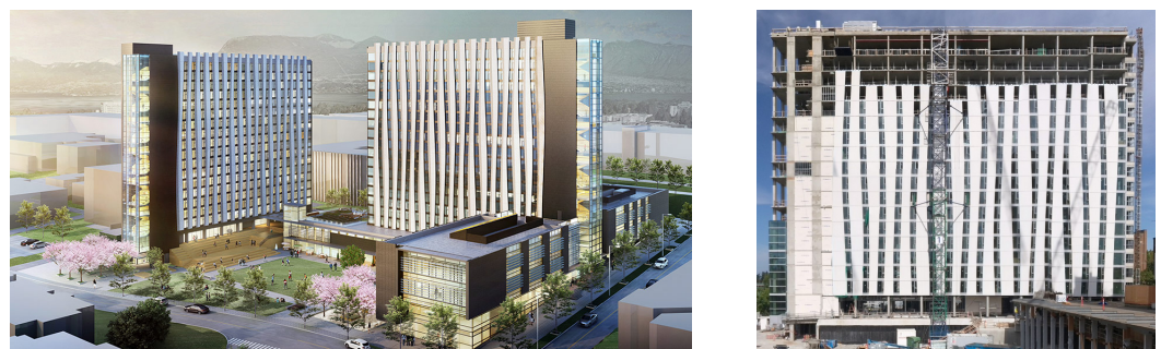
Figure 2. Architectural design concept before the computational design for constructability (left) ©Perkins+Will; Constructed façade after the computational design for constructability (right) ©BIM TOPICS Lab.
