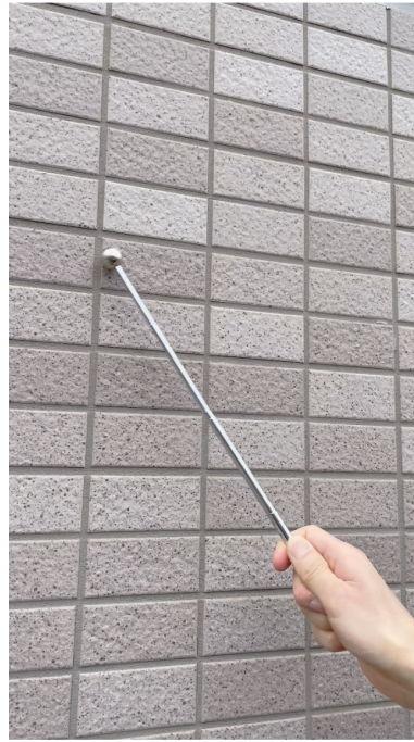
Figure 5. Hammering test on a tile wall (rubbing the surface).
