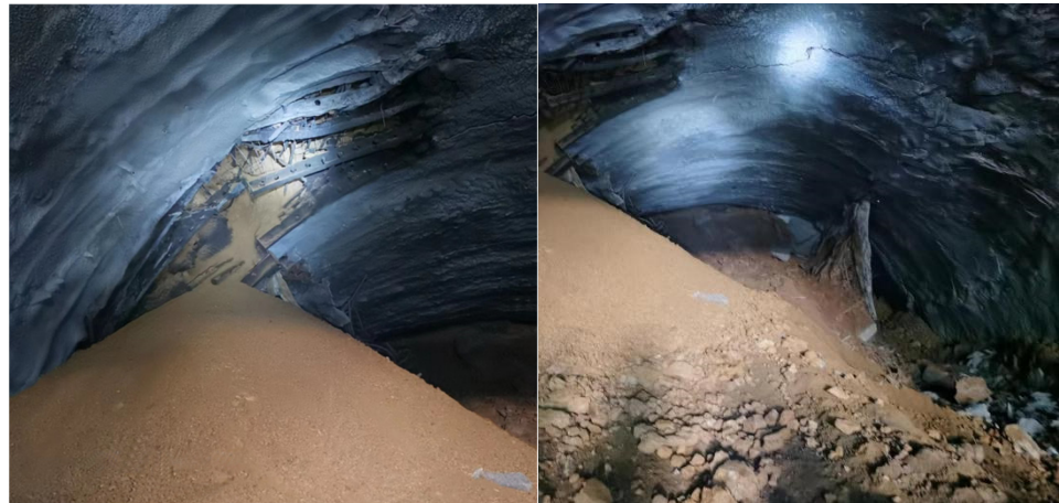
Figure 11. Section 1 of the landslide accident. Section 2 of the landslide accident.
