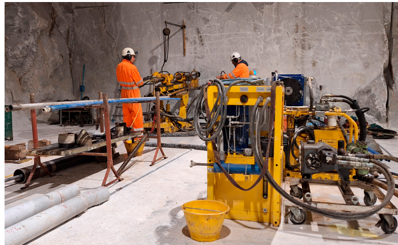
Figure 6. Stages of a sub-horizontal borehole drilling.
