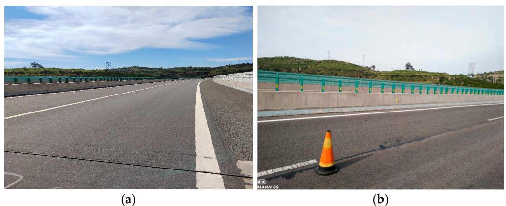
Figure A2. Disease observation of deck pavement, guardrail, and sidewalk: (a) deck pavement has no disease; (b) guardrail and sidewalk have no disease.
