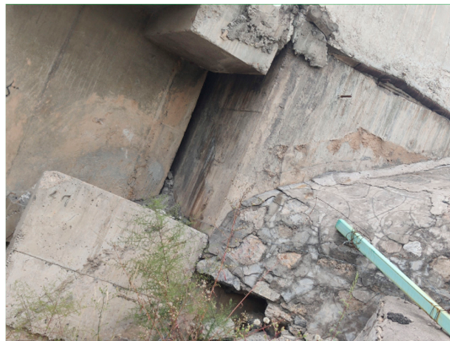
Figure A7. Wing wall and ear wall are basically intact.
