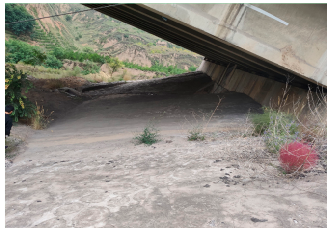
Figure A8. Cone slope and slope protection are basically intact.
