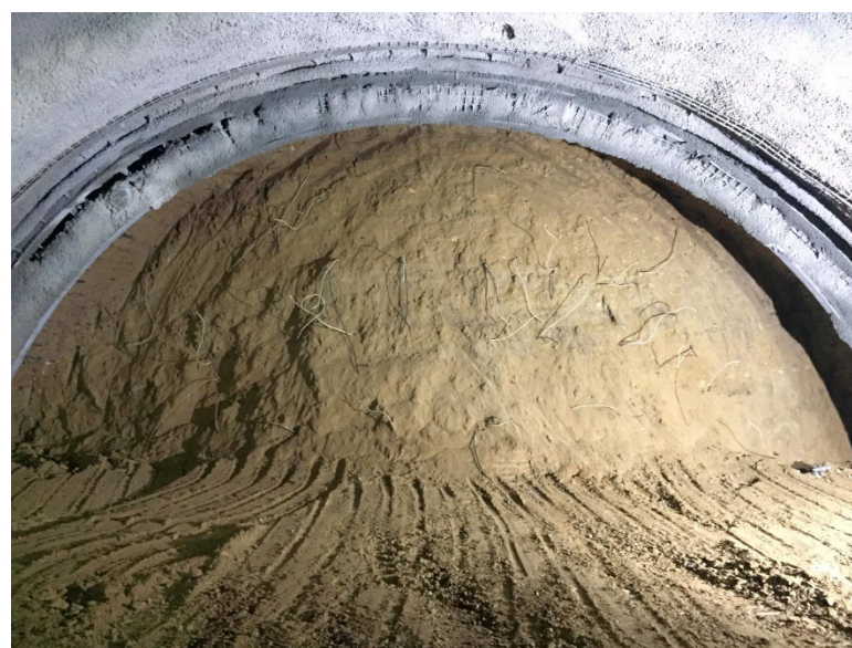
Figure 23. Tunnel excavation face.
