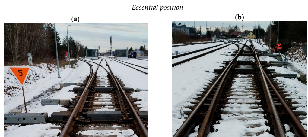
Figure 10. View of turnout No. 12 from the beginning (a) and end (b) of the turnout.
