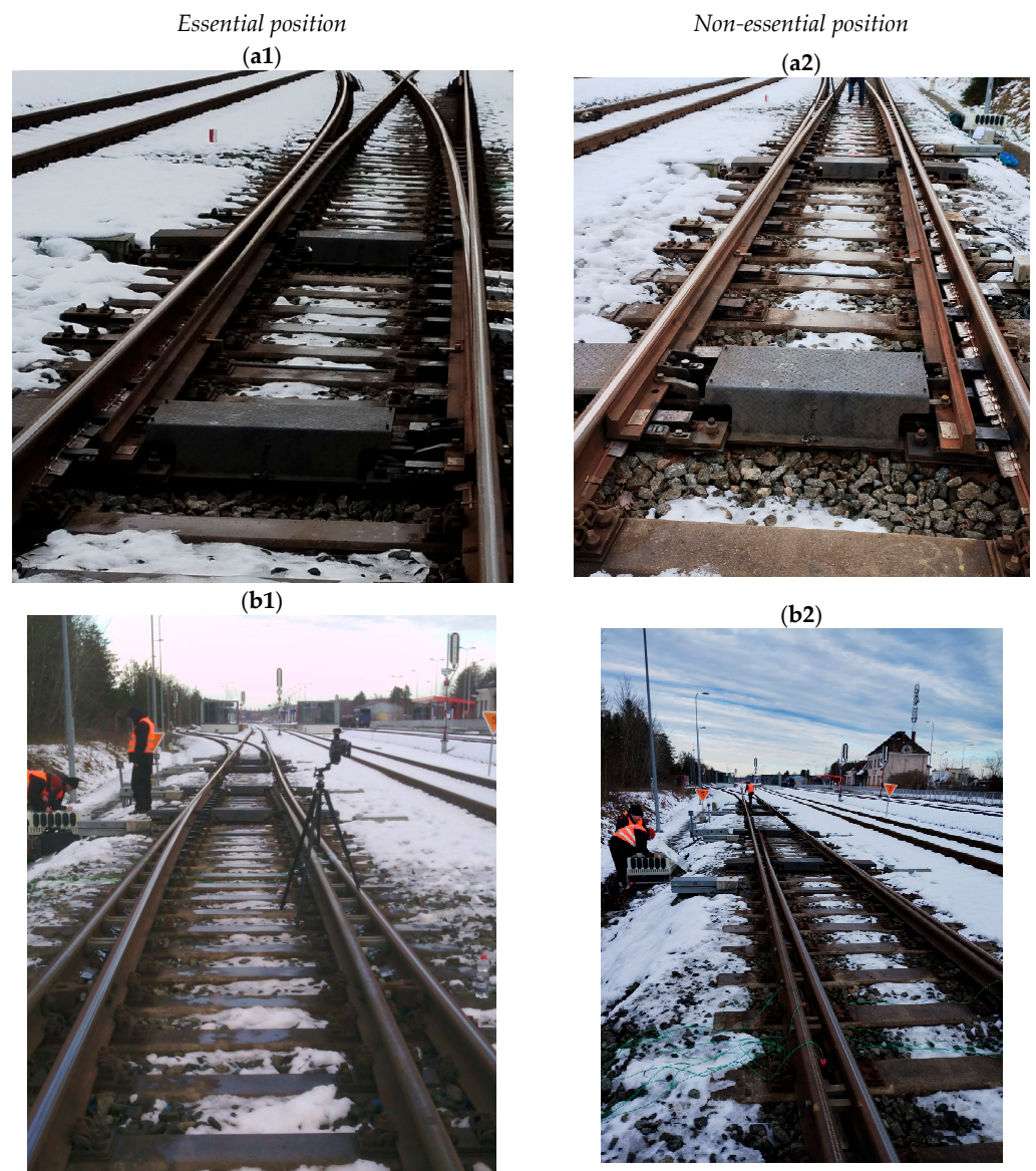
Figure 9. View of turnout no. 11 from the beginning (a1,a2) and end (b1,b2) of the turnout.
