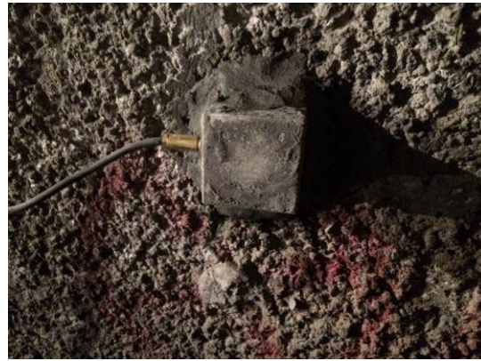
Figure 2. Sensor bonded to the lining of the tunnel.
