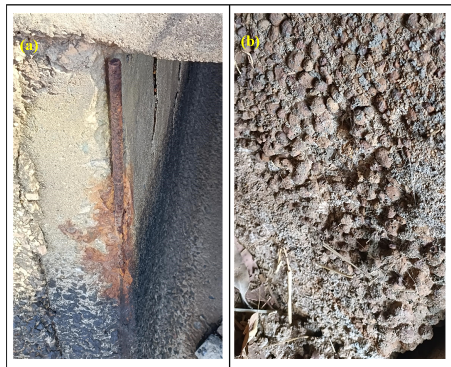
Figure 6. (a) Low clear cover and (b) round-shaped aggregates observed in some cases.
